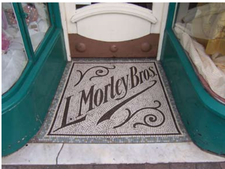
A good example of a recessed doorway, with level access.
