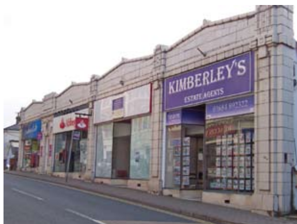
Existing inappropriate fascia hiding original features and destroying the street scene
