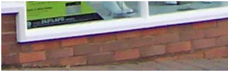
Example of a Modern brick stallriser
