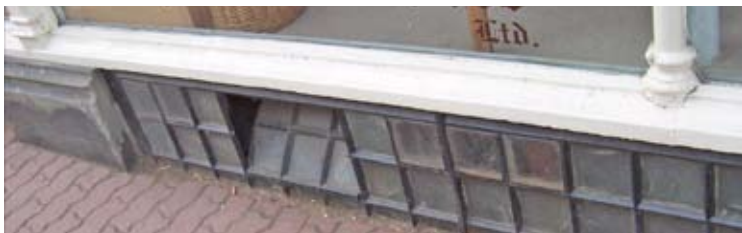
Example of glass blocks stall riser, 1920's.
