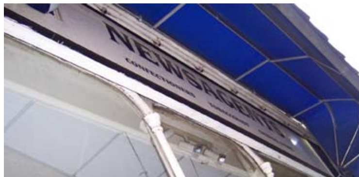
Oversized fascia concealing the ornate window frame and a canopy blind concealing the fascia
