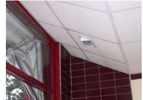
The above photograph shows a false ceiling raked from the window
