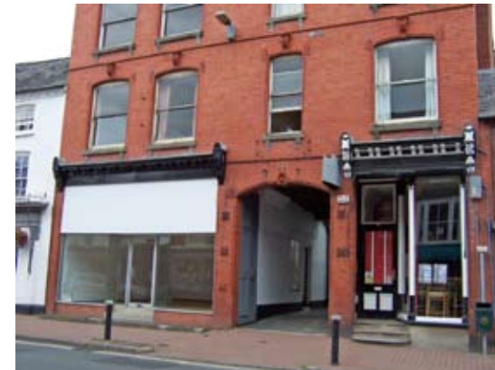
Examples of an oversized fascia
