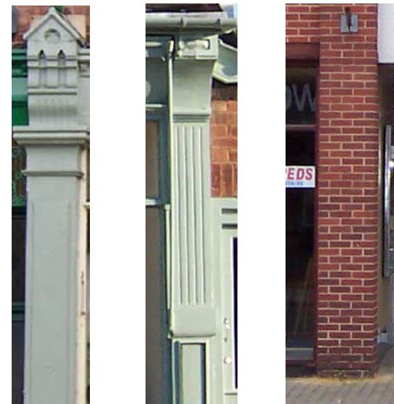
A stone, timber and brick pilaster
