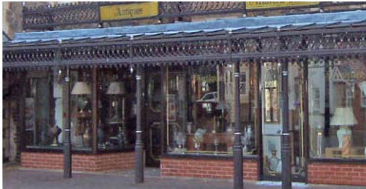
An example of a canopy integrating with shop front design.
