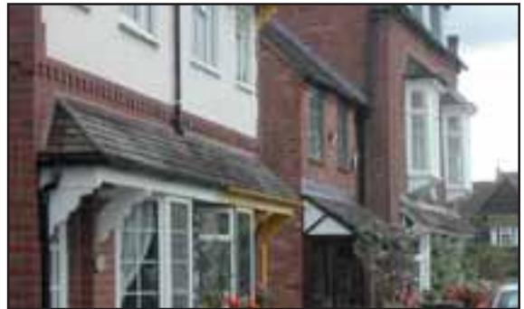
Tiled weatherings replicated on traditional and modern dwellings.
