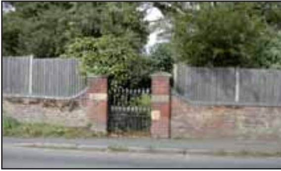
Traditional pedestrian gate in Main Road.
