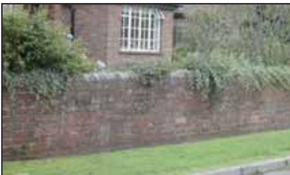
A brick wall close to the crossroads with bull nosed bricks.
