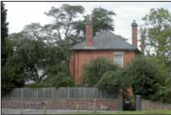
This Victorian building emerges into view.
