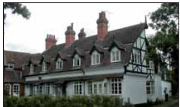
Lea Cottages with its unusual gambrel roof.
