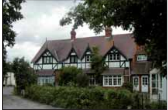
Lea House makes a positive contribution to the area.
