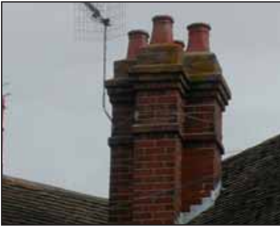
Distinctive tall chimneys.
