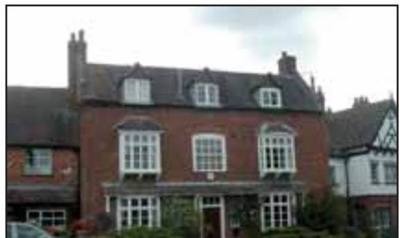
Traditional brick on Post Cottage.
