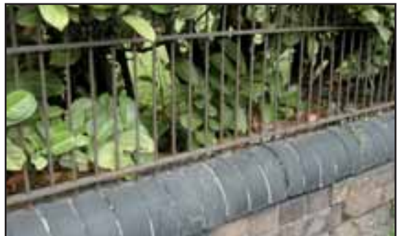
Boundary walls a feature at the crossroads. Note the original railings.
