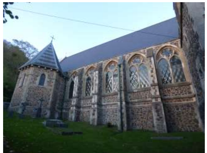
The banded slate roof and latticed windows at St Wulstan's church
