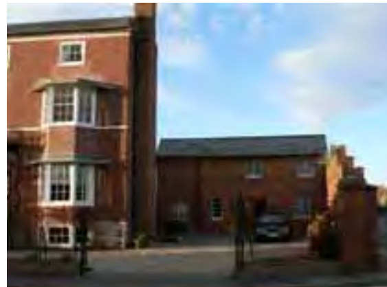
More sympathetic extensions being sensitively subservient, featuring sensitive materials with regards to bricks and roof along with good fenestration pattern
