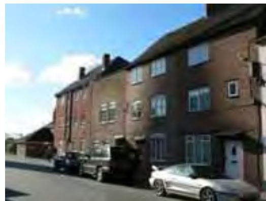
New build sympathetic in scale and massing but not in its detailing.
