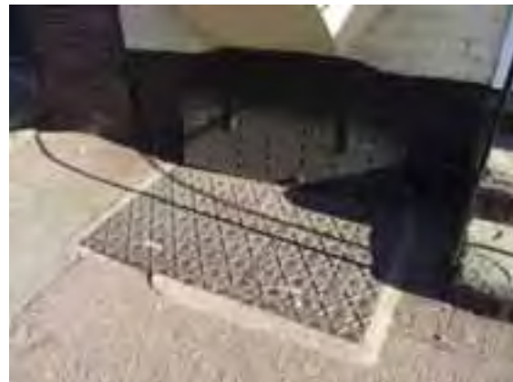
Cast Iron Cellar doors on Old Street
