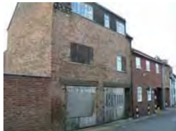
Negative building in Court Row
