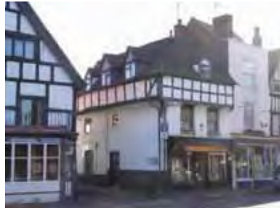
Jettied floors on High St
