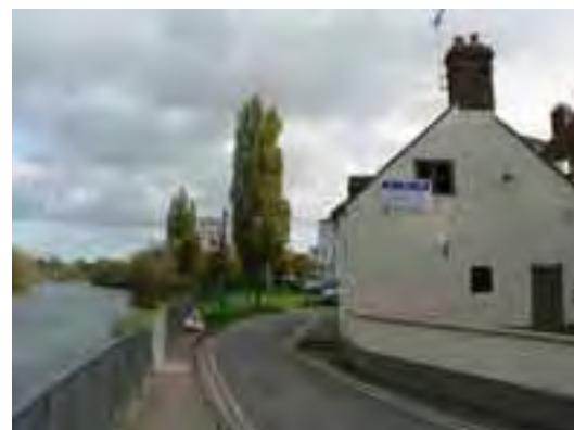
Unattractive fencing along Waterside
