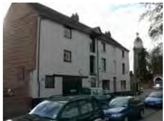
Looking south west along Waterside
