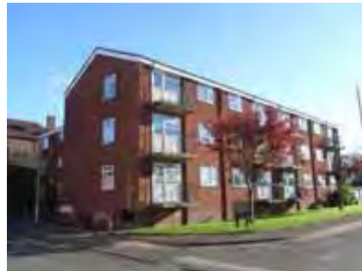
Unsympathetic new build
