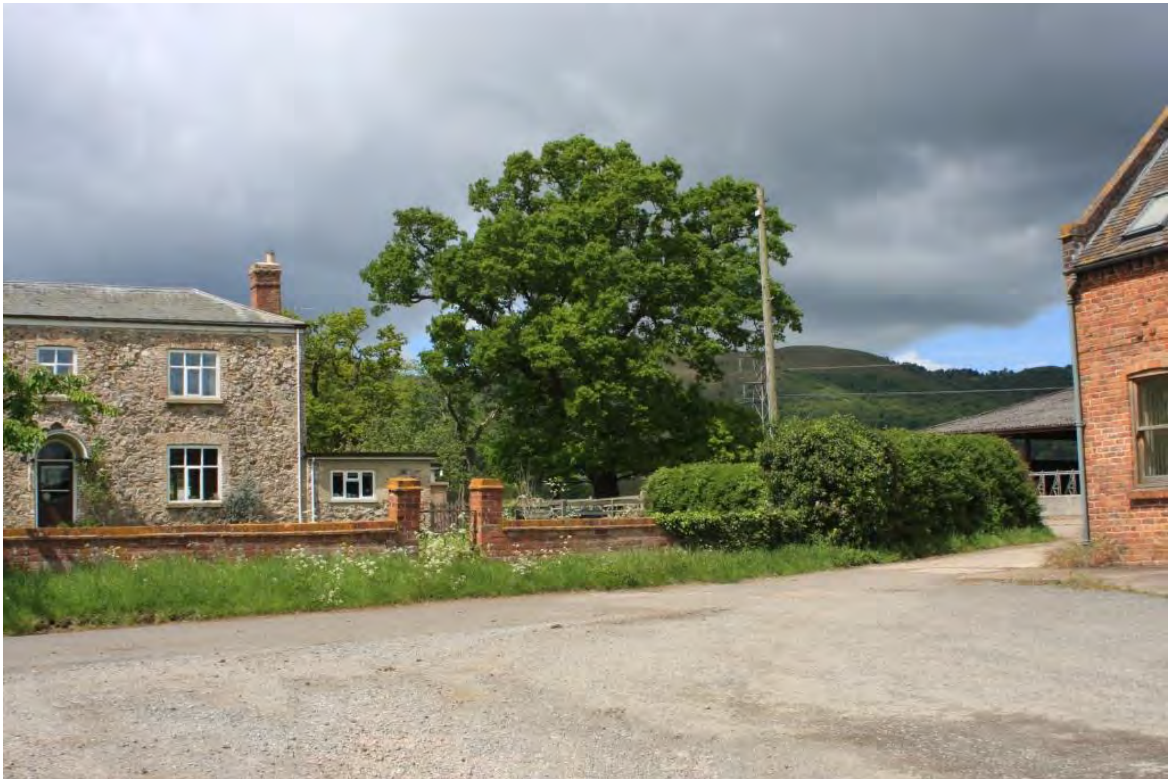
Wood Farm looking north west towards Malvern Hills
