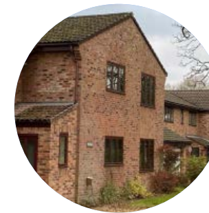
Multi-tonal bricks, corbelling and porches
