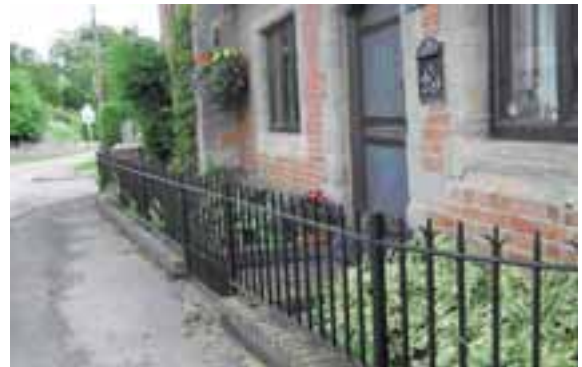
Railings and metal gate at the Forge
