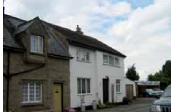
New addition with differing roof pitch and wide first floor windows
