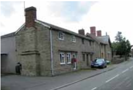
Removed boundary disrupts the line of the street
