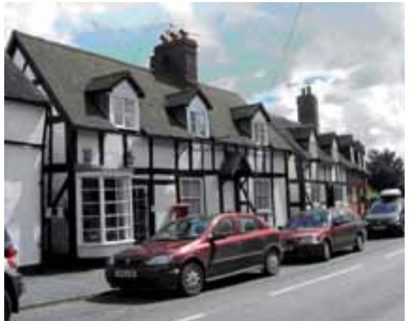
Timber framed with inserted dormers...
