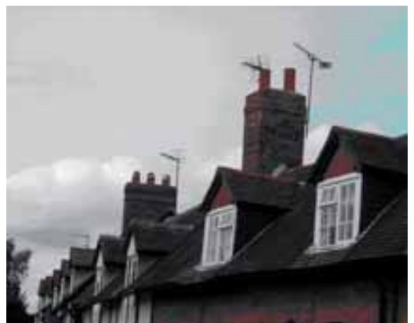
Typical dormers and chimneys. Note how the earlier dormers on the timbered buildings begin at roof plate level.
