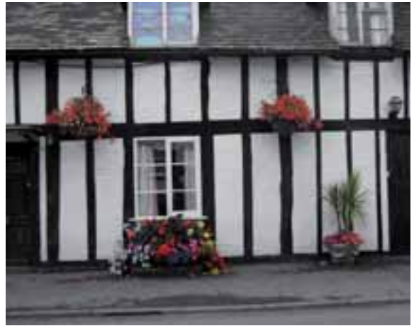
Closely framed cottage with simple casement windows.
