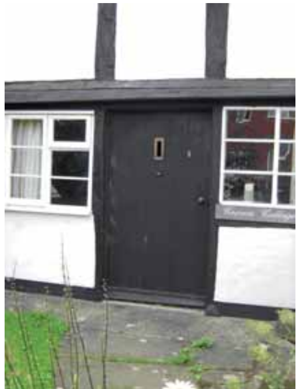
Traditional boarded door
