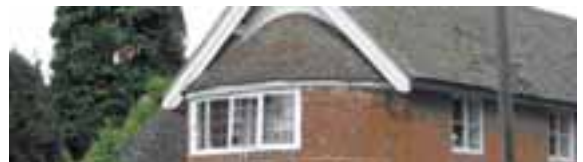
Plain tile roof at Kenelm Cottage.
