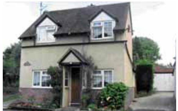
An infill property with widened and upvc fenestration.
