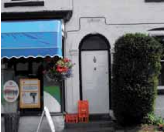
Early C19 door and door surround
