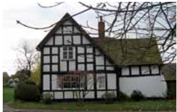
Timberframing at Bury's Place
