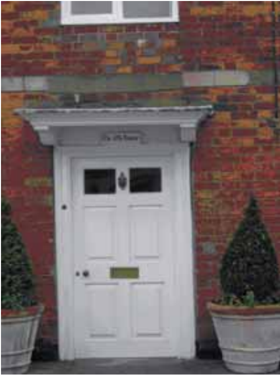
C19 door and doorcase
